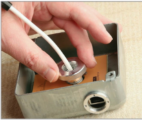
Fig D. Install the threaded nut with shoulder side down and secure.
