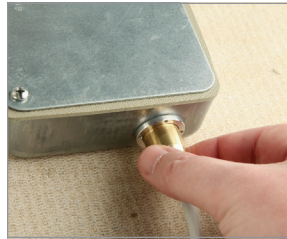
Fig H. If using Audix Cat 7 LSOH interface cable 8 , screw on the brass bell housing over the RJ45 connection and reset ceiling tile.
